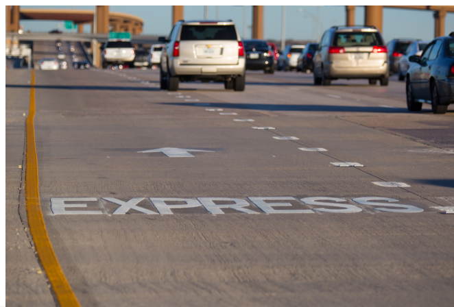
The Managed Lanes division created new roads in Dallas, Texas
